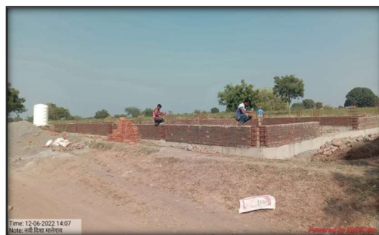
Godown construction in Progress
